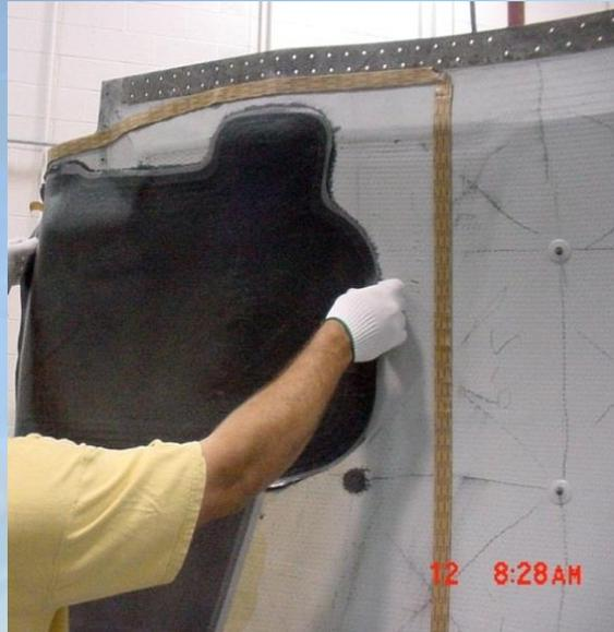
Placement of consolidated repair kit, onto structure
