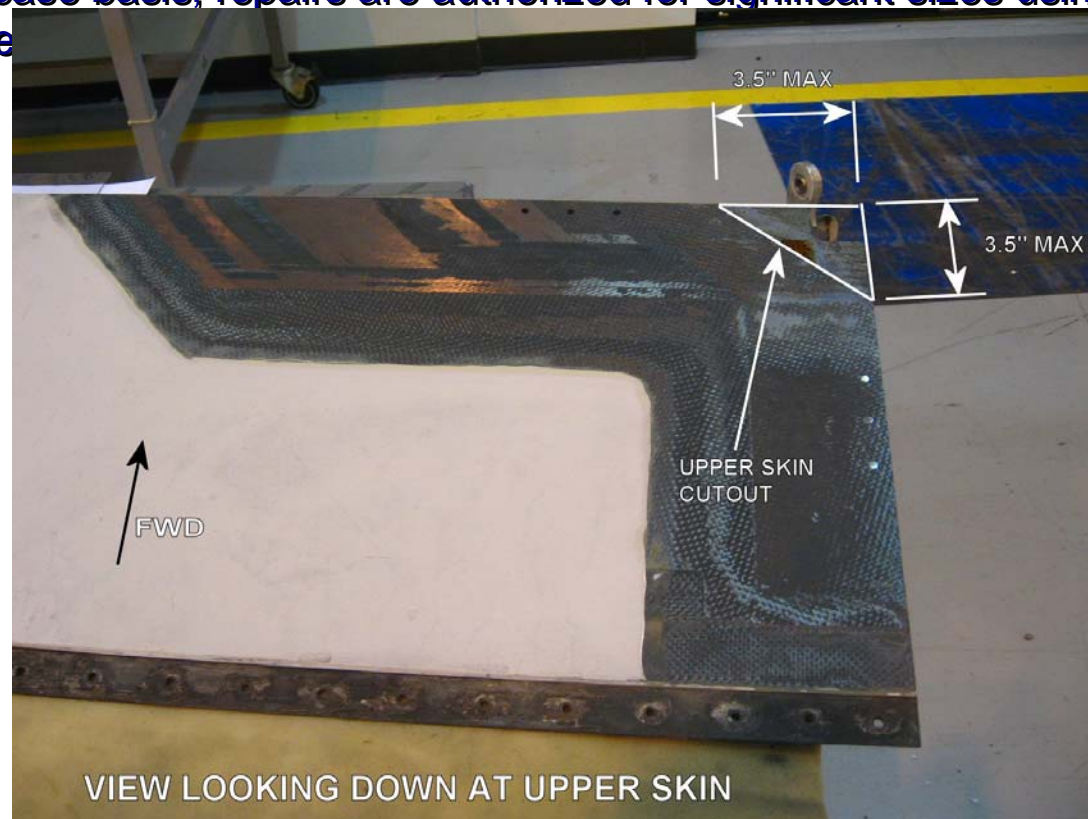
Airline Perspectives on the Constraints of Bonded Repair Size Limits
