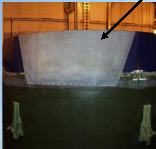
Large Area Trans-Sleeve Repair
