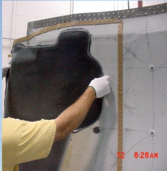
Placement of consolidated repair kit, onto structure
