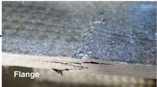
Low visibility of C-frame cracks located away from impact
