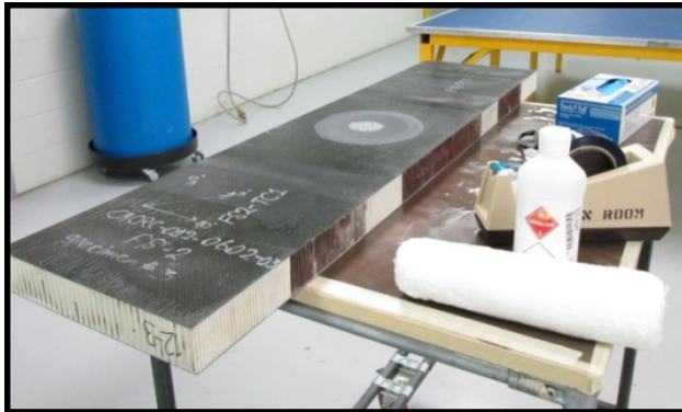
Element scarf sanded in preparation for repair
